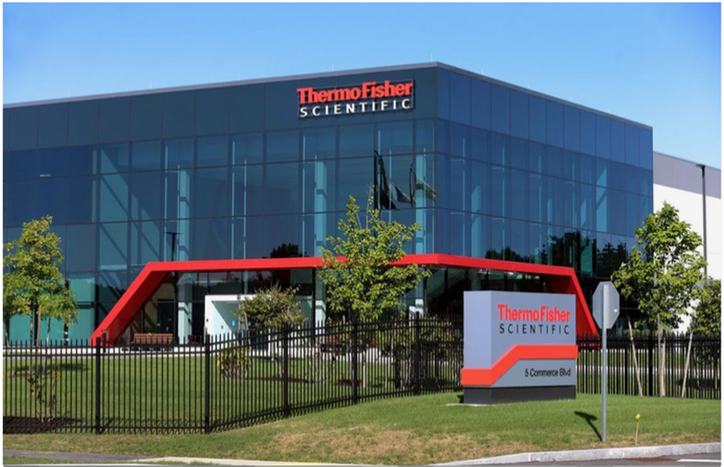
The Plainville plant is Thermo Fisher's fifth viral vector manufacturing facility. JOHN TLUMACKI/GLOBE STAFF
